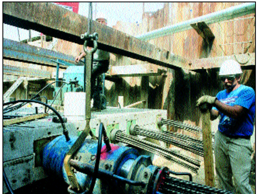
▶ At right one of the 14 tendons is tensioned in creating a total force of 8,000 kips. VSL's anchor system was used.
