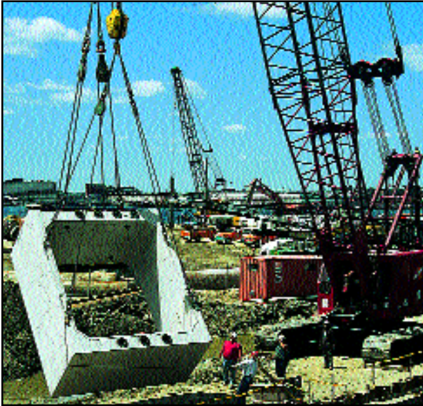
◀ Each 14' wide piece had to be tripped as it was lifted from the trailer
