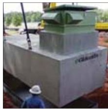
Controlled Environmental Vaults (CEV)
